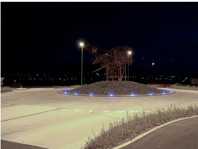
CircLED roundabout Bachenbülach
